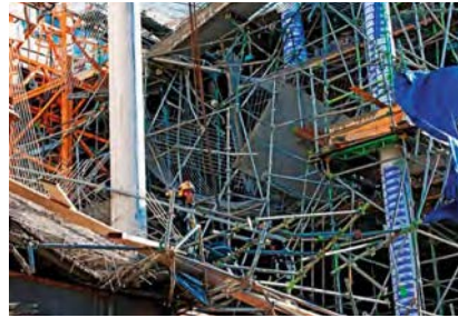
Fig. 2. Collapse of a shopping centre under construction due to an unstable scaffolding system
