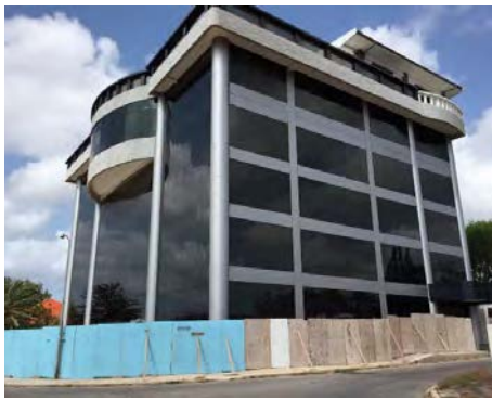
Fig. 6. Building to be investigated, Curacao 2014
