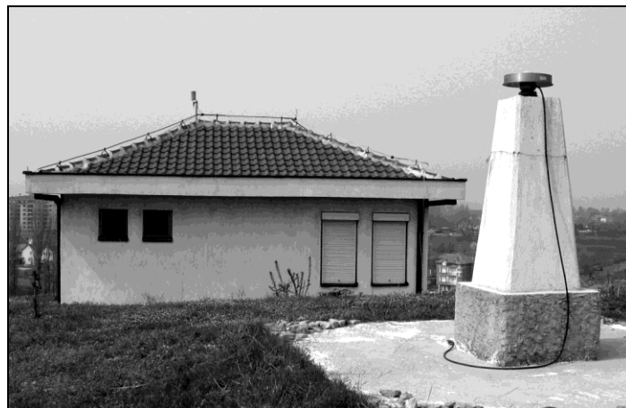
Fig. 4.6.2.3. Permanent GPS station in Ohrid
