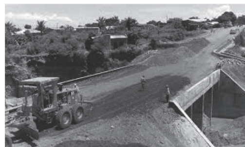
Fig. 1. Road construction site, Bujumbura rural [4]
