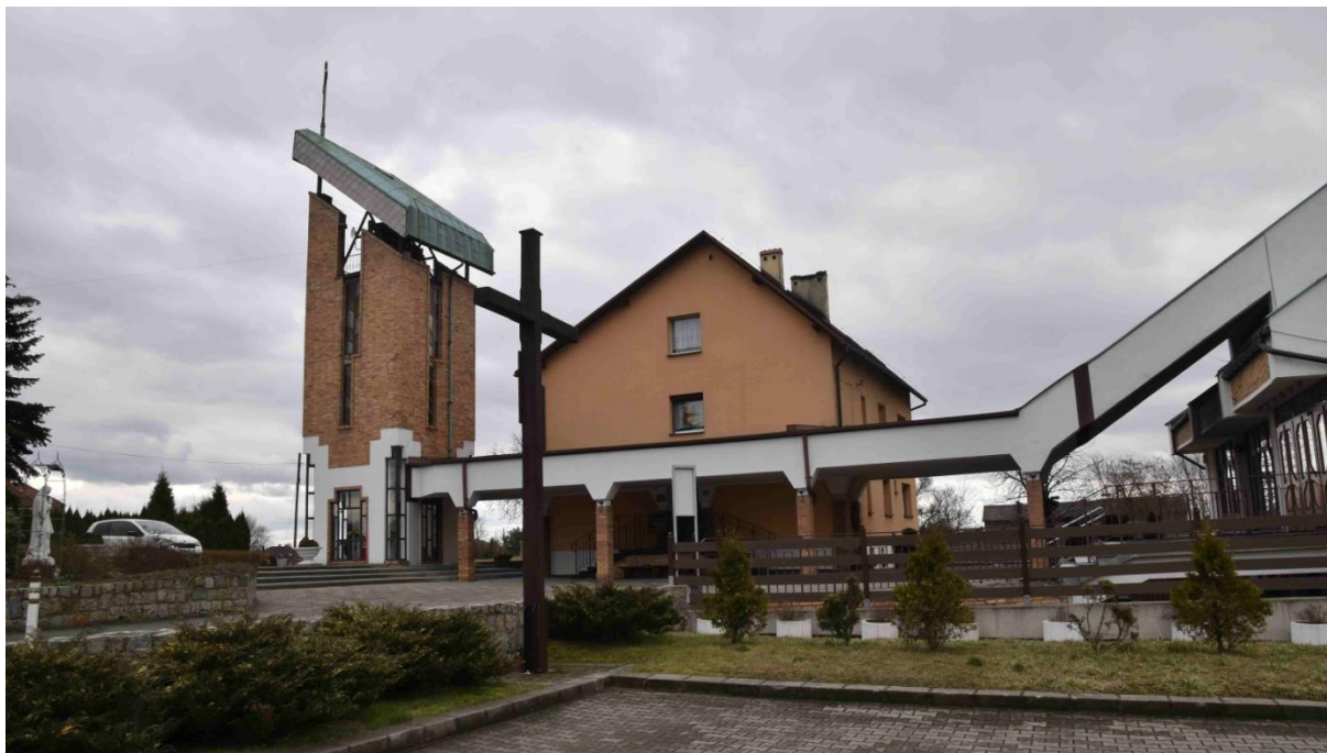
Fig. 3 Structure A of the testing ground - bell tower, parish buildings visible in the vicinity
