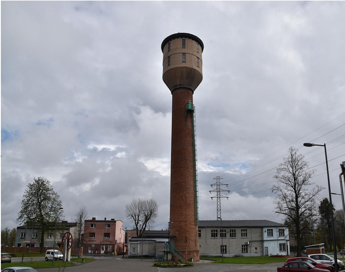
Fig. 5 Structure C of the testing ground - view of the viewing tower after the rehabilitation of the industrial water tower
