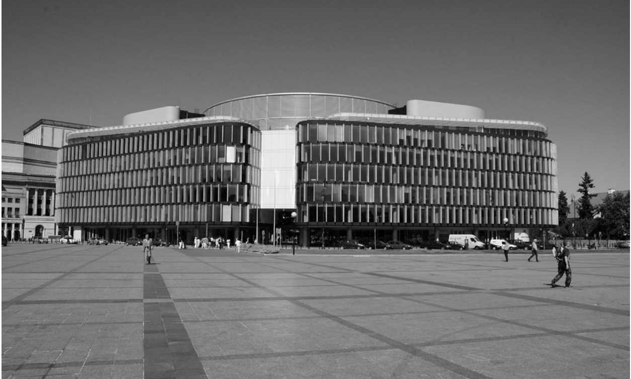
Fig. 1. Norman Foster, Metropolitan Building, Piłsudski Square, Warsaw, 1997-2003, a) View from Piłsudski Square, b) courtyard; photo: A. Szczebrzeszyński
