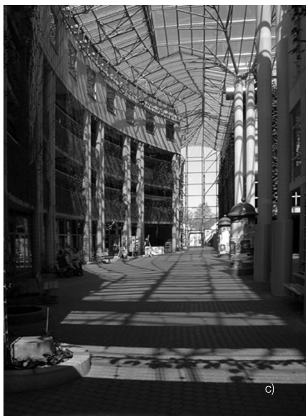
Fig. 4 a,b,c. Marek Budzyński, Zbigniew Badowski, Warsaw University Library (facade, vestibule, catalog room) Warsaw, 1993-1999; photo: M. Budzyński
