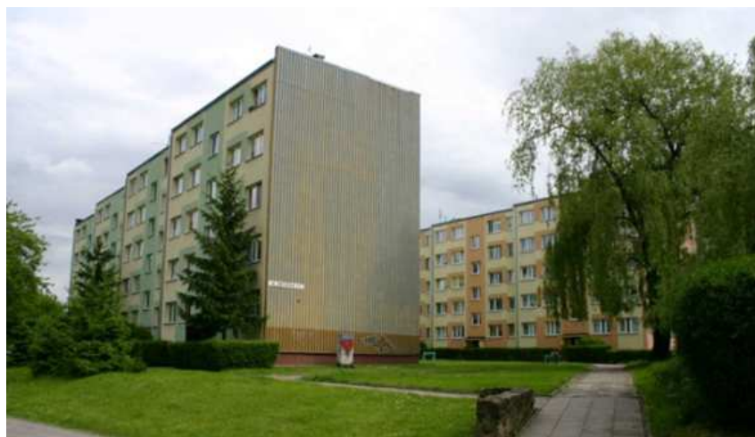
Fig. 5. Leśnica, prefabricated houses in Snycerska and Majchra streets, Phot. A. Kononowicz, 2009
