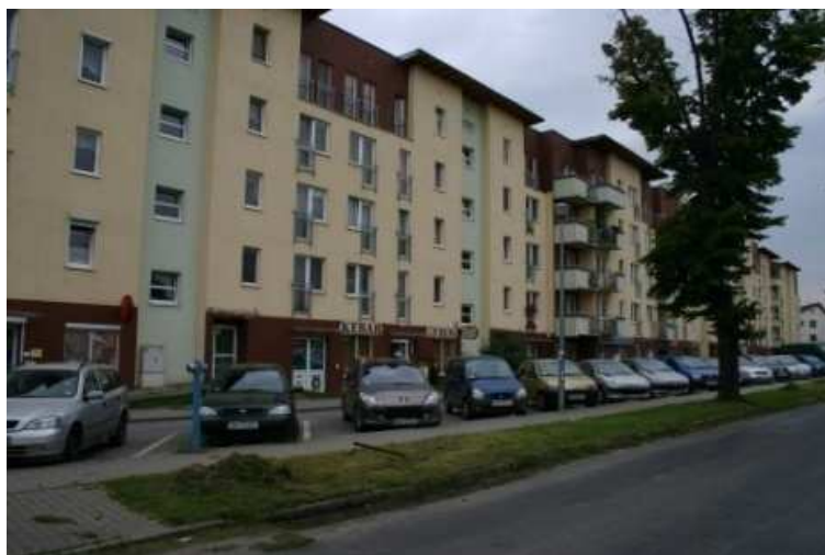
Fig. 7. Buildings along Dolnobrzeska Street, Phot. A. Kononowicz, 2009
