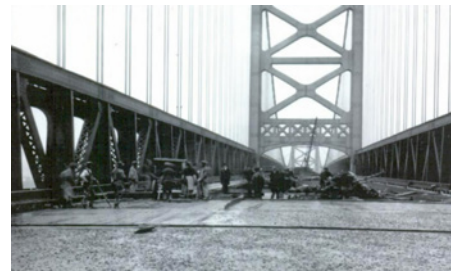
Budowa mostu Camden (Benamina Franklina), fot. Delaware River Port Authority Archive
