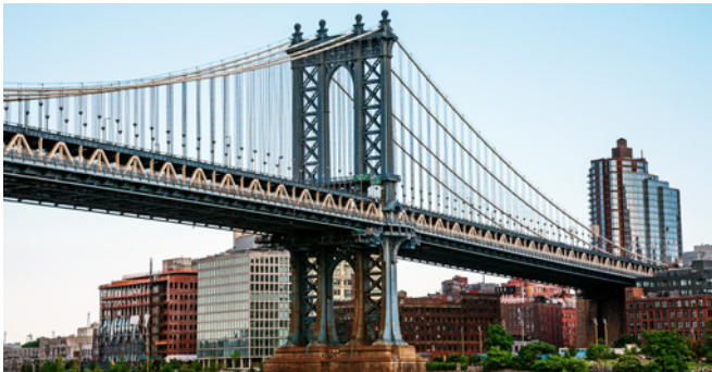
Pylon i kratownica mostu Manhattan, fot. Mohit, Adobe Stock
