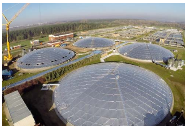
Figure 3. Primary settling tanks after hermetization
