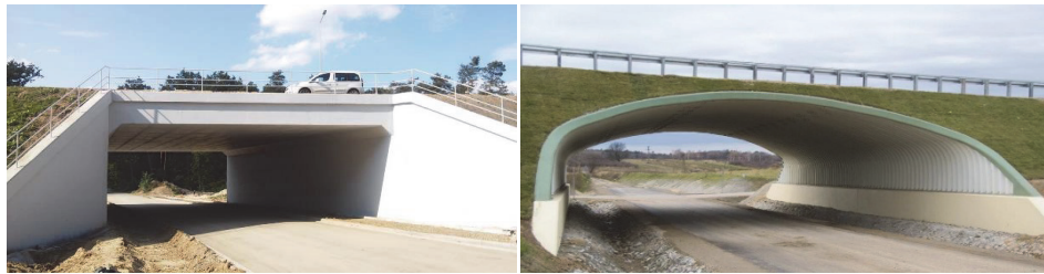
Fig. 6. Two bridges having the same function – a) concrete, b) buried corrugated steel bridge
