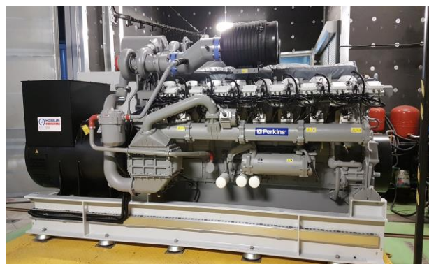
Fig. 5. The Perkins 4016-61TRS2 industrial gas engine is equipped with the specially developed system hydrogen-methane fuel system. The genset arrangement at Horus-Energia test facility
