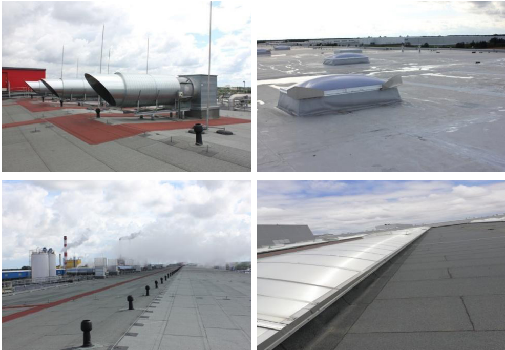
Fig. 1. Crucial areas in flat high-volume rooftops. Source: B. Ksit
