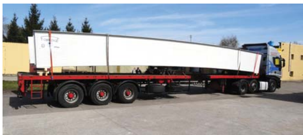
Fig. 11. Transporting the footbridge span
