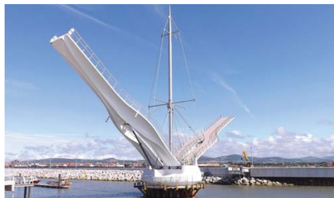
Fig. 4. The drawbridge Dragon's Bridge in the port of Rhyl in Wales [www.gurit.com]
