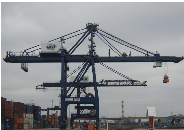
Figure 1. The container gantry crane
