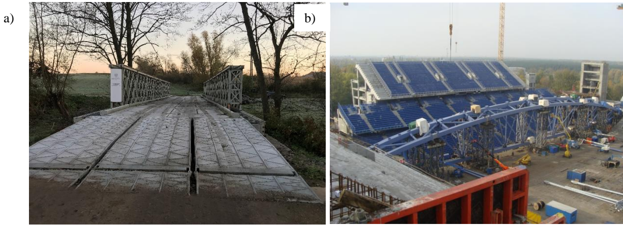
Fig. 1. Examples of the use of panel structures, a) liquidation of the effects of natural disasters - DMS 65 bridge - Szeligi near Płock (2021), b) L-36 bridge structure as support scaffolding for the lattice girder of the Poznań stadium roof (2011).
