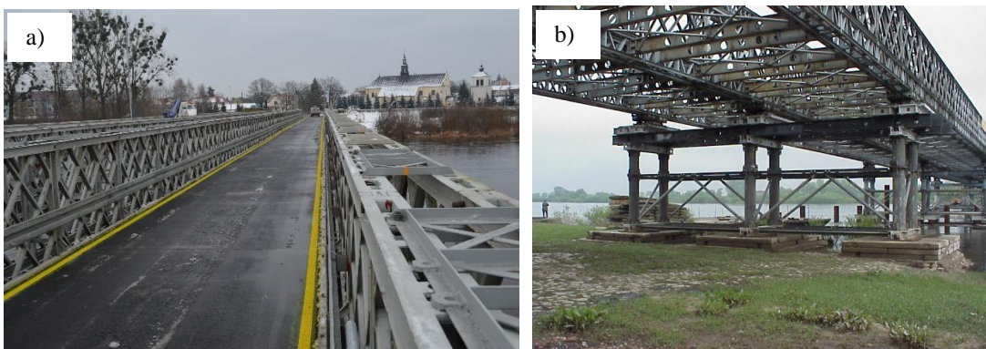
Fig. 2. Use of military collapsible bridge structures as diversion structures, (a) Ostrołęka bridge (2017), (b) Kiezmark bridge (2002).
