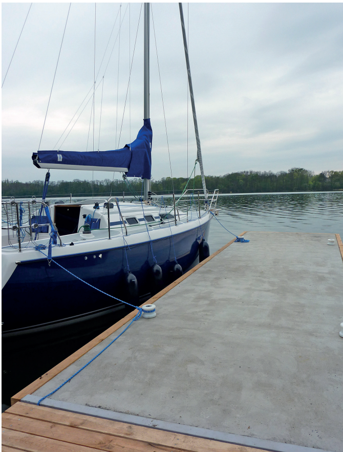
Fig. 13. View of the commissioned pontoon with the platform
