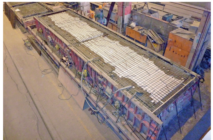
Fig. 10. Concreting of the upper plate of the pontoon
