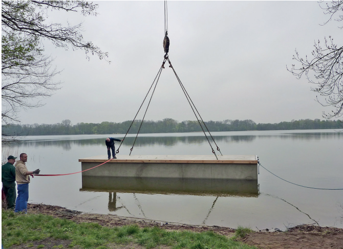
Fig. 12. Launching the pontoon
