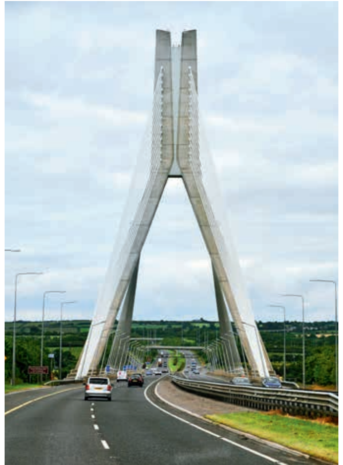
Ryc. 25. Pylon mostu Mary McAleese Boyne Bridge
