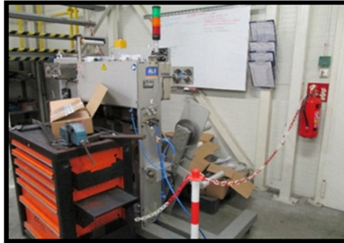
Fig. 4 Area before implementation of the 5S method
