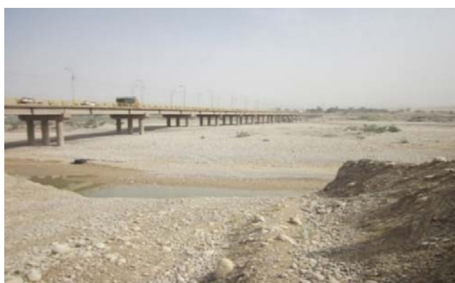
Photo 1. A view of Sardasht Zeydun bridge on the Zohreh River at upstream of the material mining zone (phot. F. Azarang)
