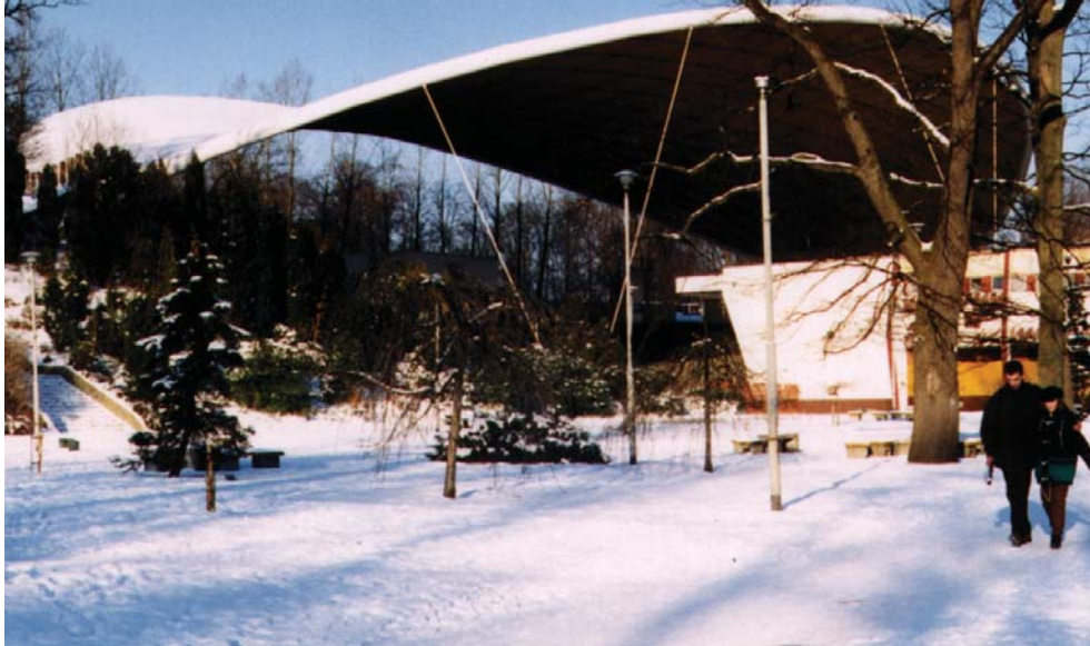
Fig. 1. The suspended roof over open-air theatre in Koszalin
