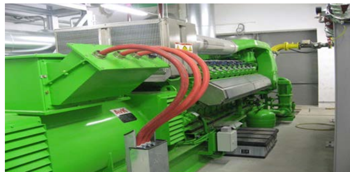
Rys. 4. Silniki gazowe EC „Wesola” (Mysłowice) [7] Pic. 4. Gas engines in „Wesola” plant (Mysłowice) [7]
