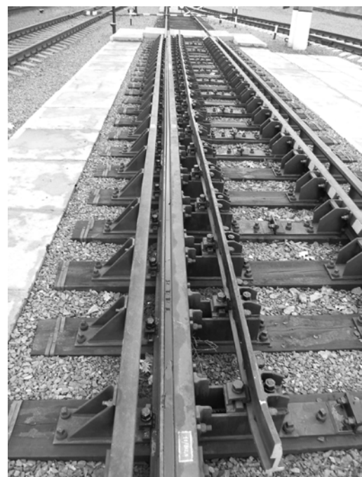
Fig. 3. Rail gauge change stand for the SUW 2000 system [28]
