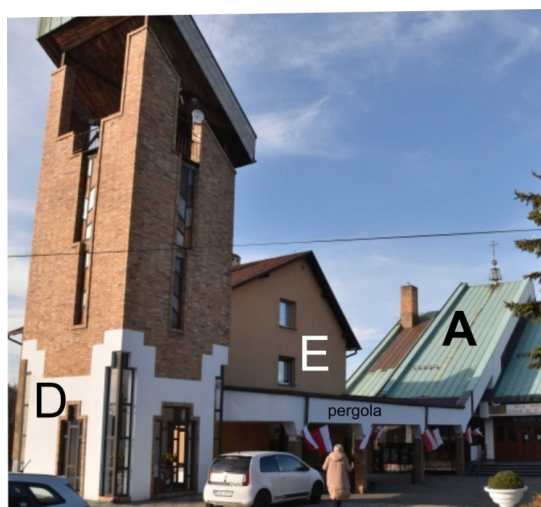
Figure 2. View of the church building and tower
