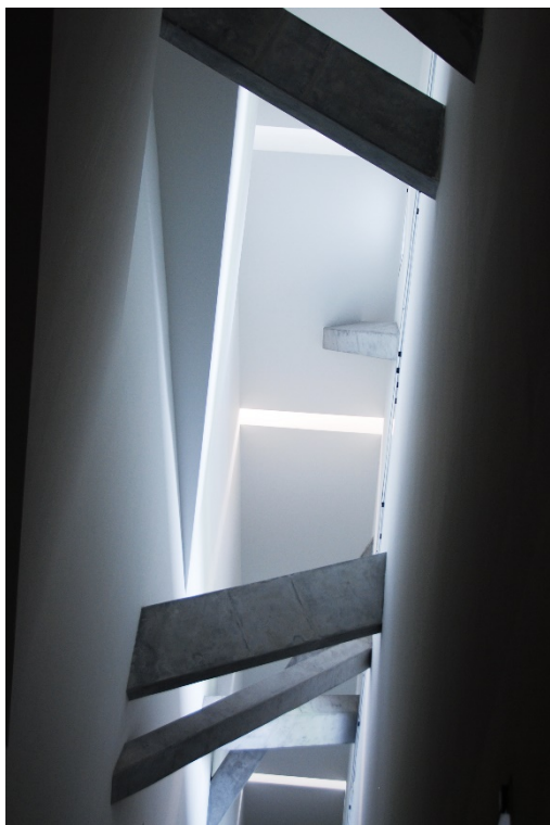
Fig. 7. The interior, lit by daylight running through small openings in the ceiling, is composed by irregular array of concrete beams. Source: photo J. Badach
