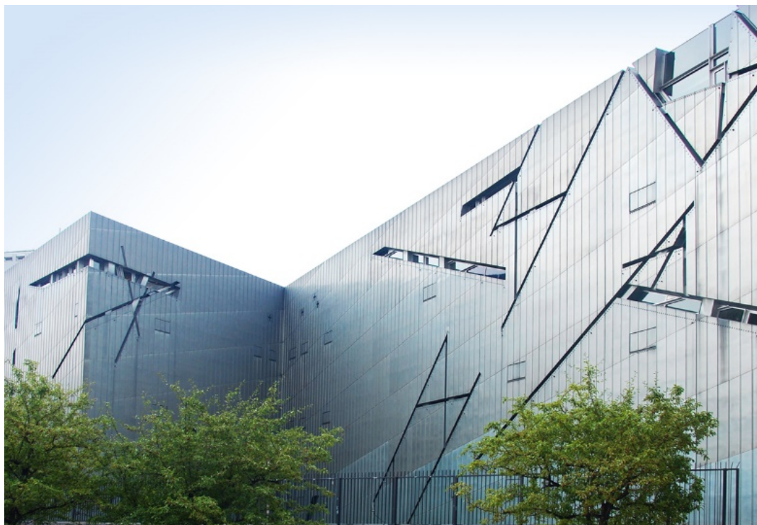
Fig. 3. The Jewish Museum façade covered with zinc panels cut by irregularly shaped glazing. Source: photo J. Badach
