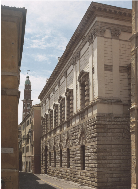
Fig. 19 Vicenza, Palazzo Thiene, The façades from Contrà San Gaetano, after the conservation and reconstruction of the plaster layers of the 1990s (Photo Credits: Christoph Ulmer)
