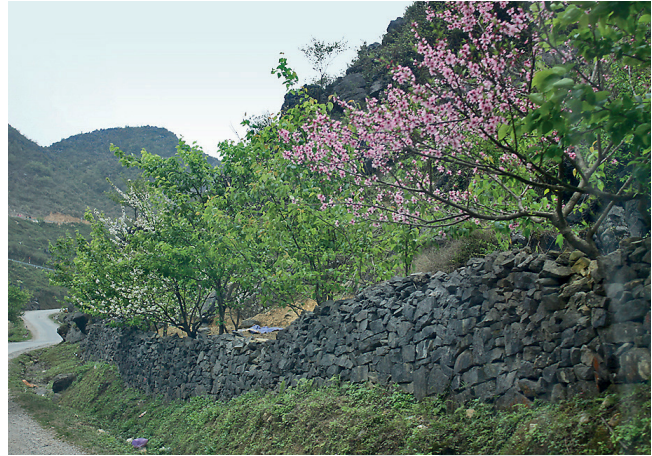
Fig. 17. The wall made of limestone in Dong Van district, photo Dao Quoc Bao
