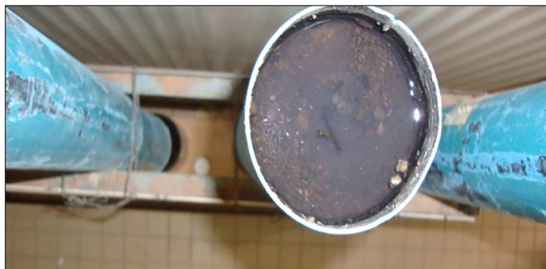
Figure 4. Filter clogging
