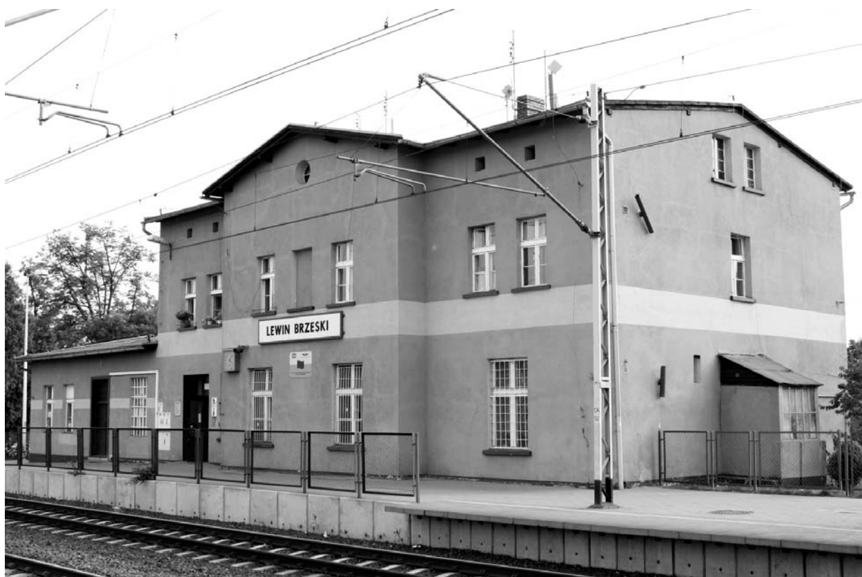
Fig. 7. Building of the station in Lewin Brzeski. During the modernization conducted in 2007 walls were covered with an even layer of polystyrene foam, due to which all details of the elevation were covered depriving the entire building of any stylistic values. Additionally, it was painted in the expressive orange colour (Pic. by author, 2009).
