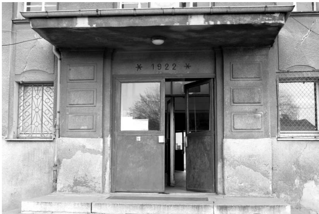
Fig. 5. Modernist door portal of the station in Olesno. Its modest geometrical detail remains in the shade of the monumental mass of the building. A characteristic extensive peak protects the wide access to the main room of the station. The door carpentry dates back to end of the 20th century (Pic. by author, 2009).
