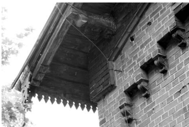
Fig. 1. Decorative carpenter's detail of the rafter framing visible on ends of the rafter and the purlin; by their decorativeness, carpenter's decorations of eaves as well as cast-iron consoles sustaining the overhang of the gable balance strict brick walls of the station in Otmuchów (Pic. by author, 2009).
