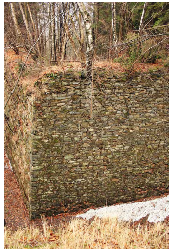
Fig. 2. Well-preserved external surface of the counterscarp wall of the fort's moat
