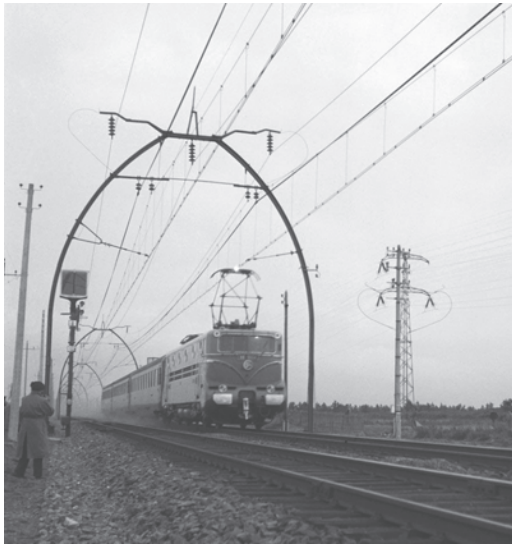
Fig. 2. Passage of a test train hauled by a BB 9004 locomotive on 29 March 1955 [source: SNCF]
