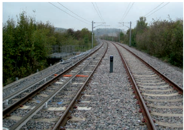
Fig. 14. Melton Rail Innovation & Development Centre test track – the left track is suitable for testing underground rolling stock powered by live rails [source: www.railway-technical.com]
