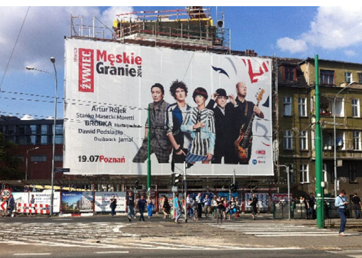
Fig. 2. Use of advertising net securing construction works (photo by M. Sylla)
