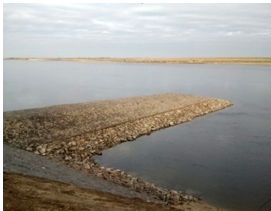
Fig. 1. Groyne on the Vistula River. Photography by the Regional Water Management Board in Gdańsk ( http://rzgw.gda.pl )
