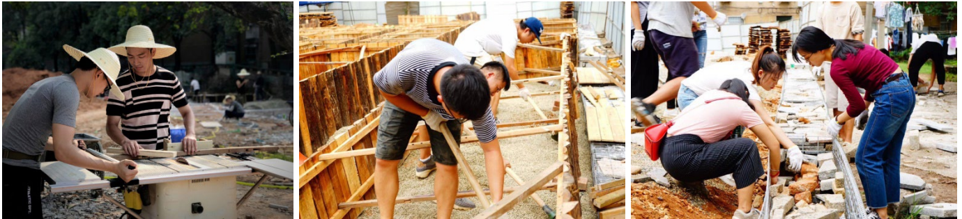
Fig. 5. Students participated to the engineering construct: a. built paths, b. built planting bed, c. built gabion (photo by Tong Li)
