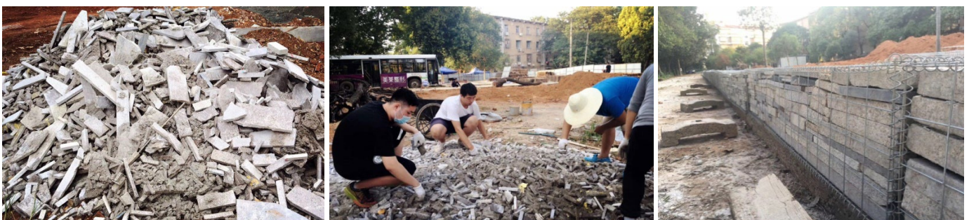
Fig. 6. The built process of the gabion: a) collect the stones, b) select the stones, c) the achievement (photo by Chen Zhou)
