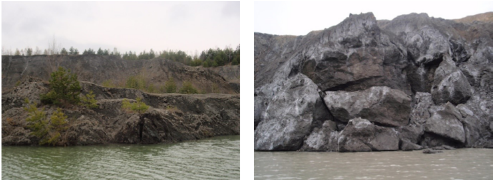
Fig. 5. Landslide and caving of the lake “Dąbrowski” shore, 2011
