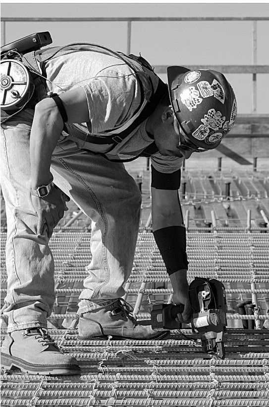
Figure 2. Tying rebar with power tier (PT).
