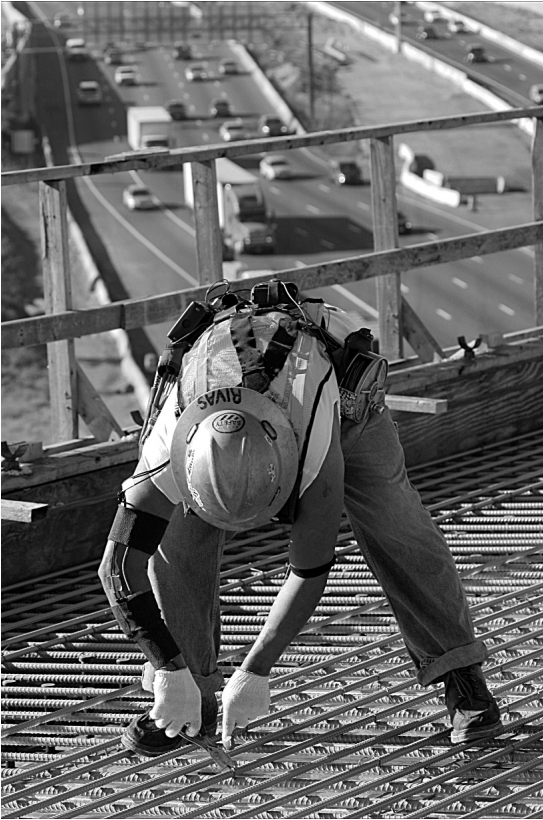
Figure 1. Traditional rebar tying with pliers and spool of wire.
