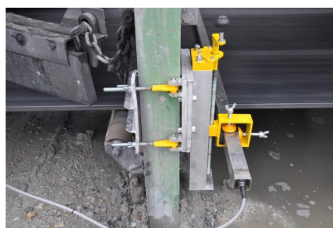
Fig. 3. Measuring head mounted in the holder to the conveyor's frame
