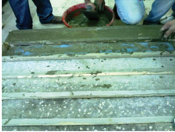
Fig. 5. Preparation of beam samples to applying the strengthening layer
