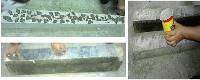
Fig. 7. Fixing the steel plate strengthening layer
