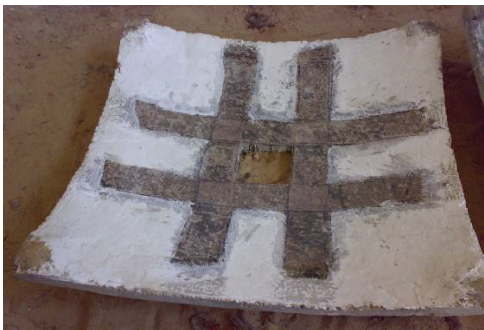
Fig. 9. Repaired shell by using 2-layers of glass fiber wrap (Type 1).
