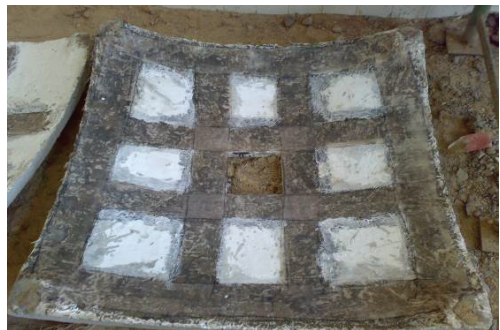
Fig. 10. Repaired shell by using 2-layers of glass fiber wrap (Type 2).
