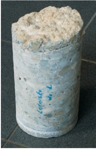
Fig. 1. A sample of the hangar slab
