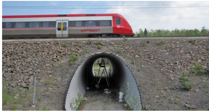
Figure 1. View of the bridge during an X52 commuter train passage
