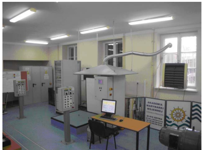
Fig. 4. Technology demonstrator of Air Independent Electric Supply System in Laboratory of Electric Drives
