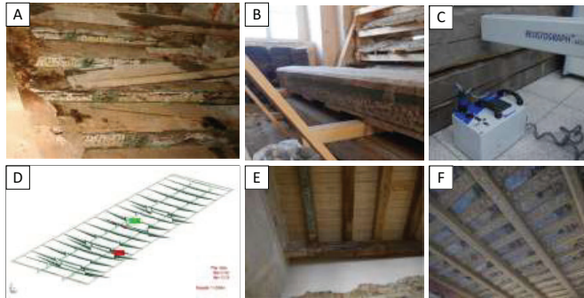
Fig. 2. Recovery of timber structural beams
