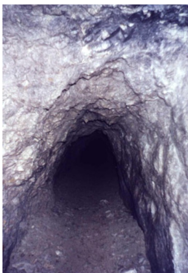
Fot. 1. Mining drift from X century, without support, developed in gneisses. Author's photo
