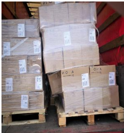
Fig. 4. Movement that significantly displaces the load behind the pallet area (own pic.)
