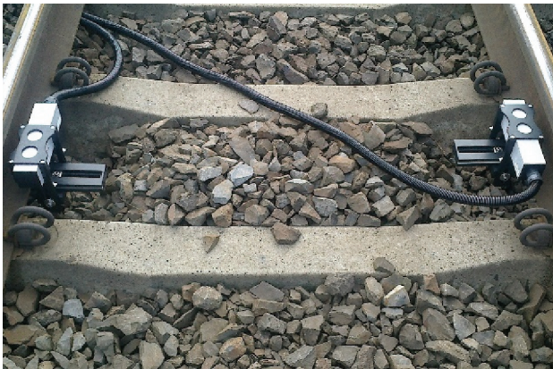
Fig. 4. Measuring antennas mounted on the railway track [Department archive]
