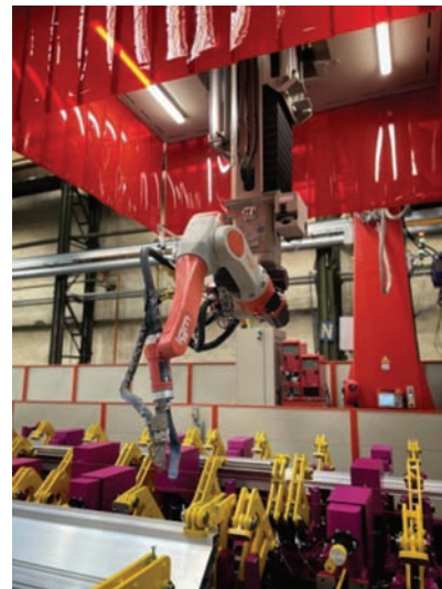
Fig. 2. Industrial robot at the Alstom Konstal plant in Chorzów [photo I. Burzyńska / Alstom]
