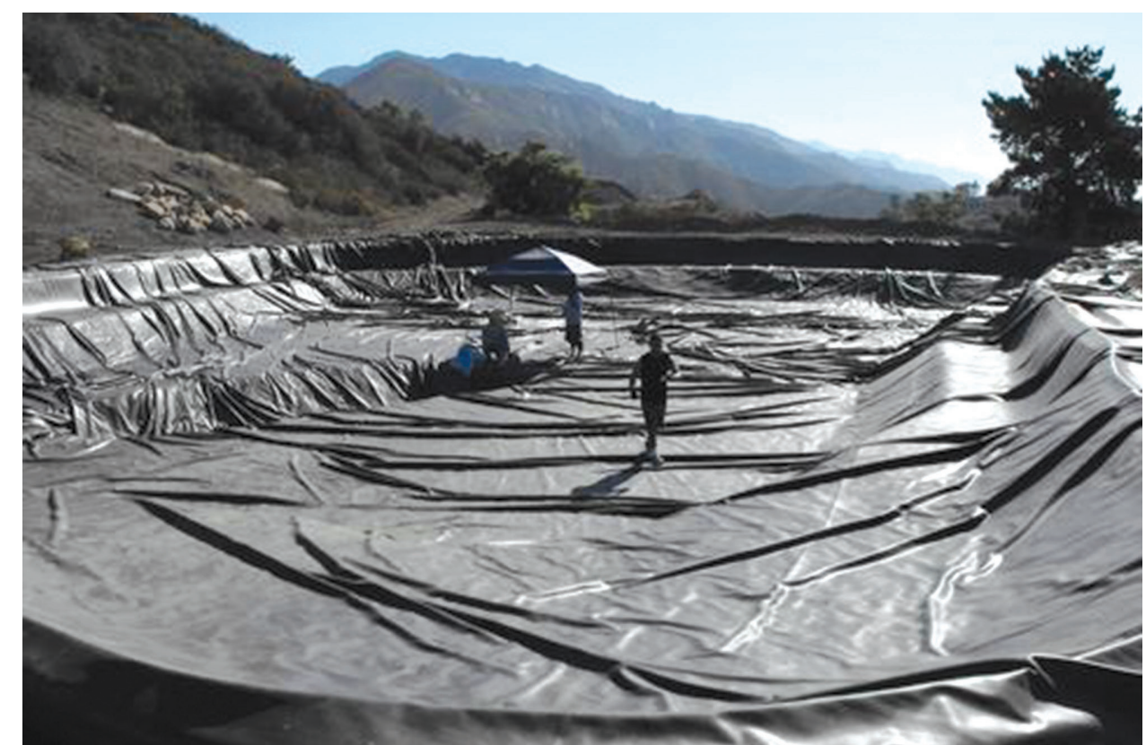
ill. 6. Organization of an artificial lake using polymeric materials in the natural landscape; https://justpondliners.com/collections/commercial-use
