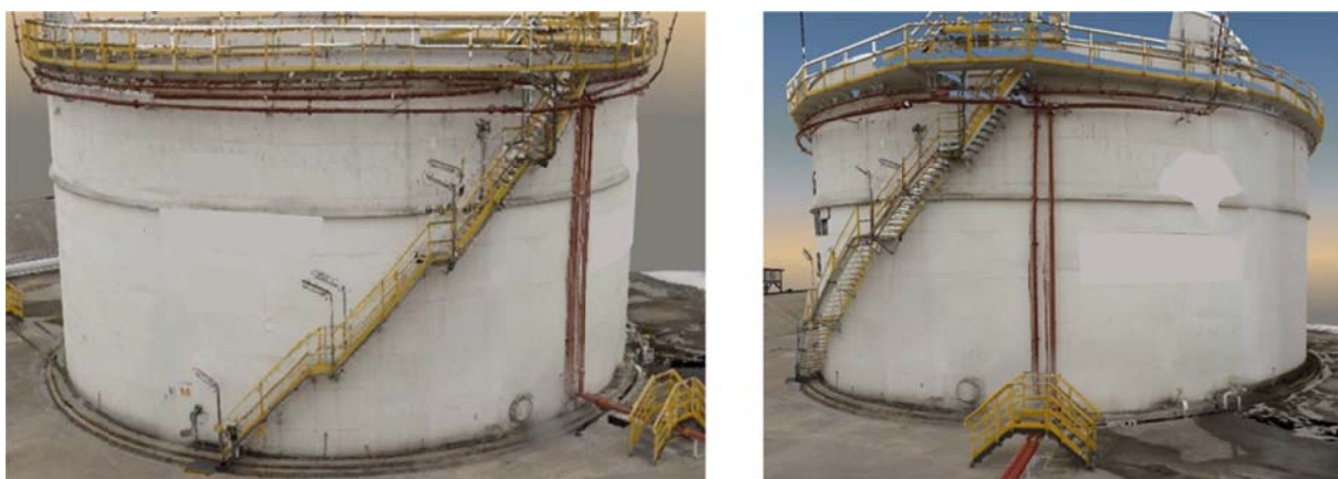
Fig.8. A point cloud acquired from terrestrial laser scanning
