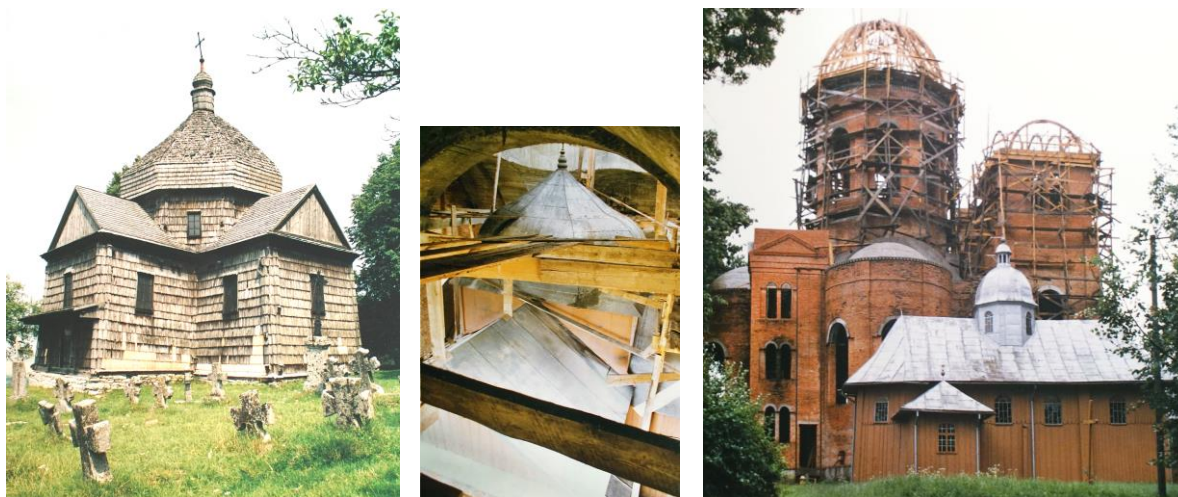
Fig. 18-20. Examples of threats to the wooden churches of Ukraine: on the left, the non-existent church in Podhorce - collapsed due to lack of proper care, in the center an old church (Chłopczyce) inside a new reinforced concrete one - waiting to be demolished, on the right - the new building displaces the still existing historical wooden building (Biskowicze). Source: photo author 1998
