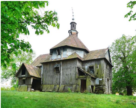
Fig. 21-22. Miekisz Stary (Poland) - an abandoned wooden church devoid of constant conservation care, northern elevation and a dome over the nave. Source: photo author 2005
