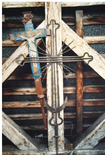
Fig. 29-30. As in churches in Poland, also in Ukraine, users - owners of church buildings - sometimes collect details that are no longer needed (?) In hiding places in bell towers. Source: photo author, 2002
