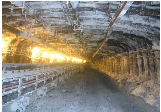
Fig. 40. Development drift secured by means of the ŁPrP variant K support
