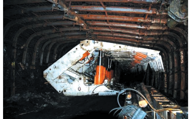
Fig. 48. Longwall equipment, development drift secured by means of the ŁPrw support
