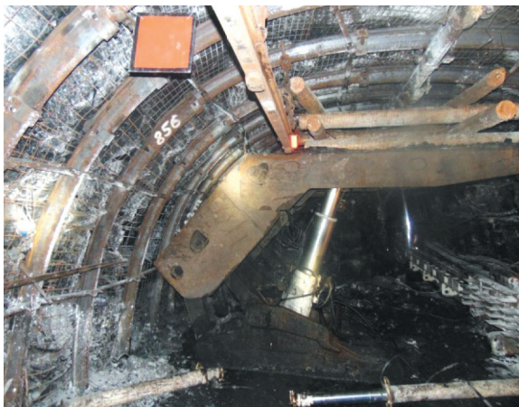
Fig. 53. Equipping a development drift driven in universal ŁPS II frames
