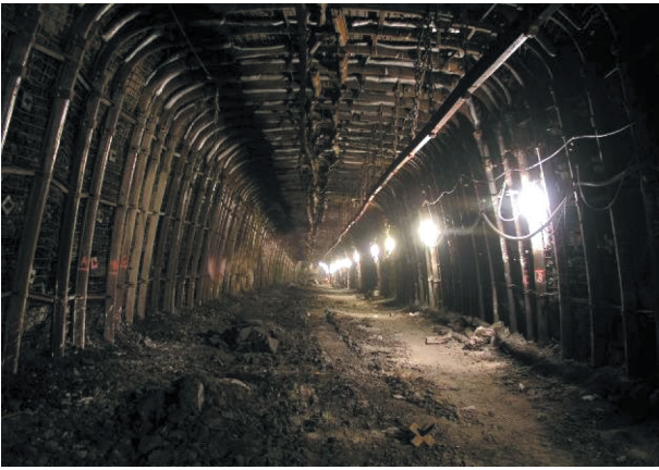
Fig. 39. Development drift secured by means of the ŁPrP variant Ł support
