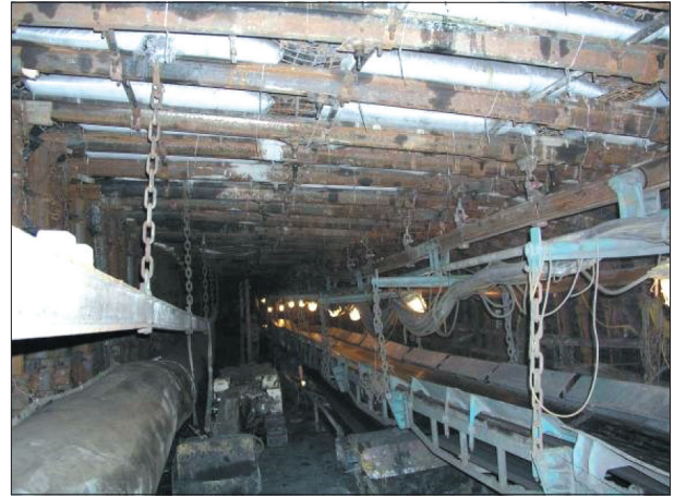
Fig. 24. Development drift secured by means of the ŁPro/A support
