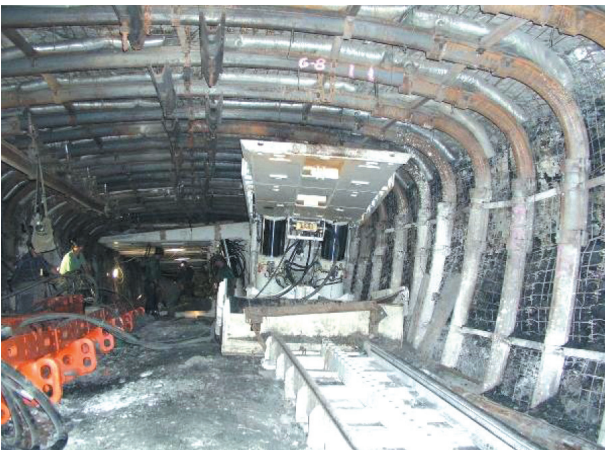
Fig. 43. Longwall equipment in a development drift secured by means of the ŁPrP variant K support
