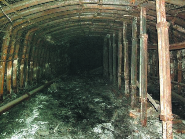
Fig. 33. Development drift secured with four-element ŁPrP frames
