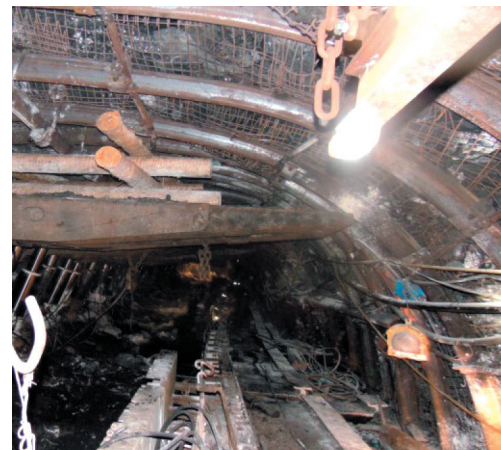
Fig. 54. Equipping a development drift driven in universal ŁPS II frames
