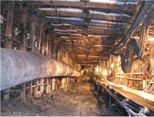
Fig. 23. Development drift secured by means of the ŁPro/A support
