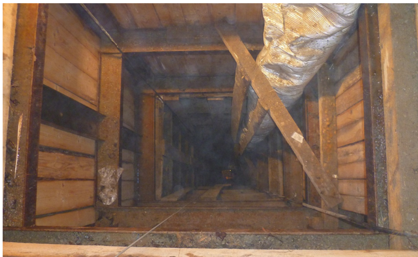
Fig. 7. View of the shaft
